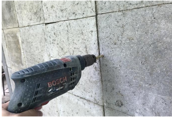
Fig. 13: Installing the developed cement boards by using screw diameter 7 mm
